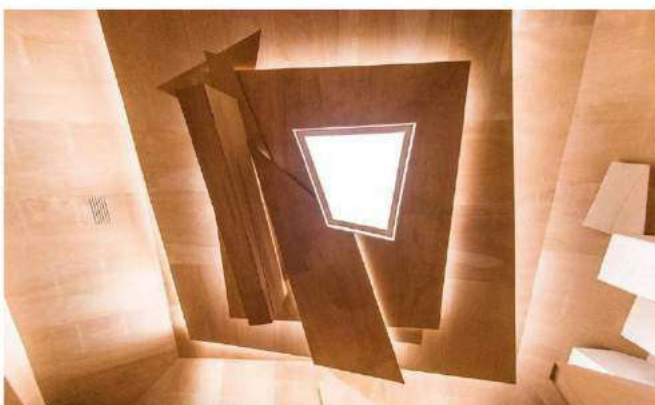
The plywood and rockwool surrounds of the French Pavilion. Photography: Giacomo Cosua
